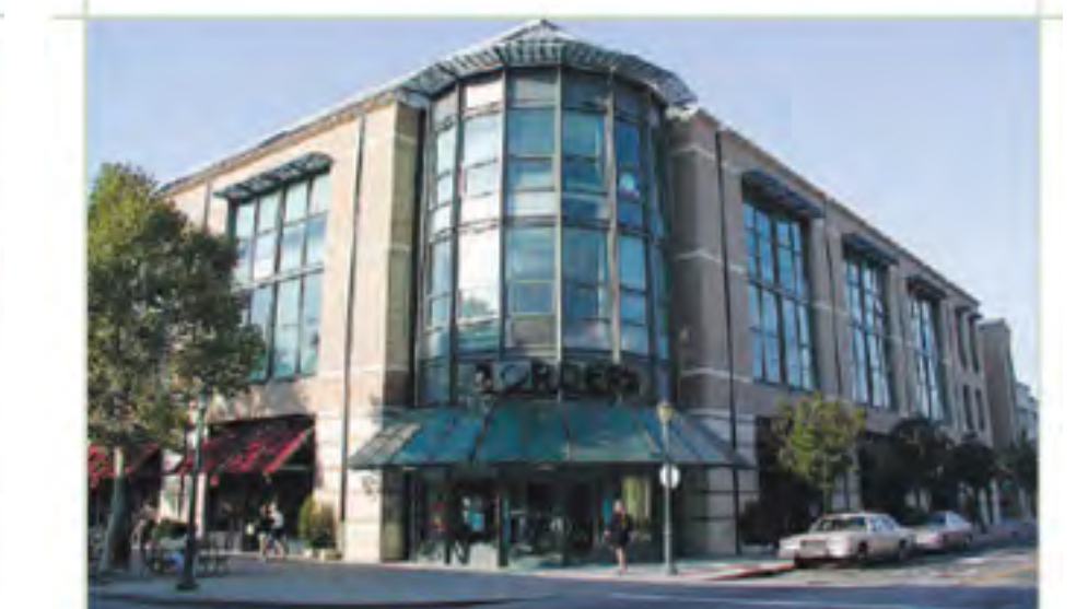
Figure 10: A prominent and inviting corner entrance.
